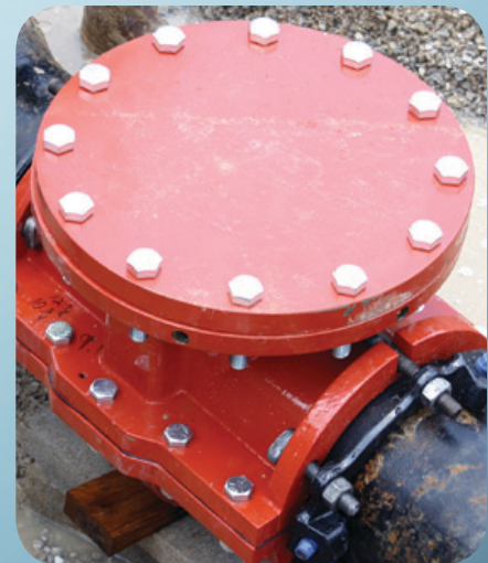
Blind flange installed.
