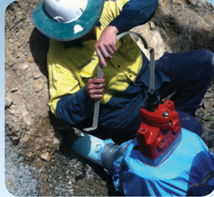
An InsertValve installation under full line pressure.
