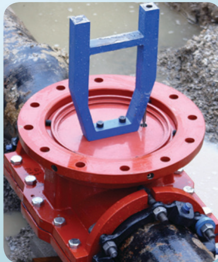
Internal equalization completion plug installed.
