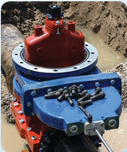
Low-profile bonnet used as line stop.
